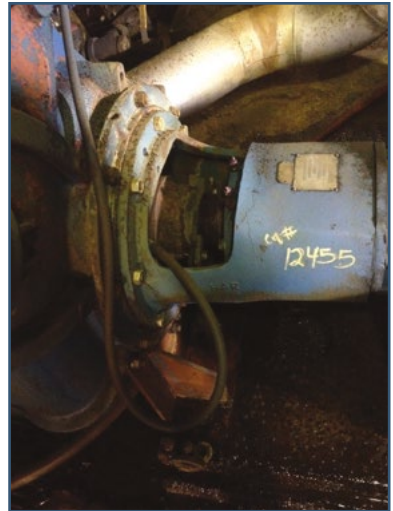
Wemco 3112 Tank Pump with SpiralTrac FIRST Device Installed
