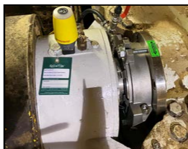
Chesterton Solution during installation and after being installed in Sulzer ZPP7 (PM5)
