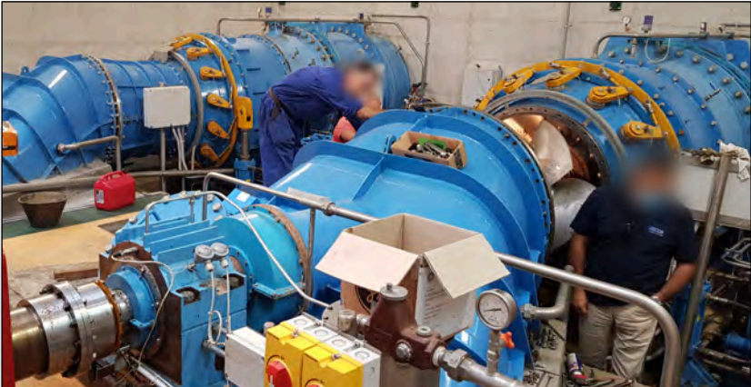
One of the Two Horizontal Kaplan Hydro Turbine being serviced
