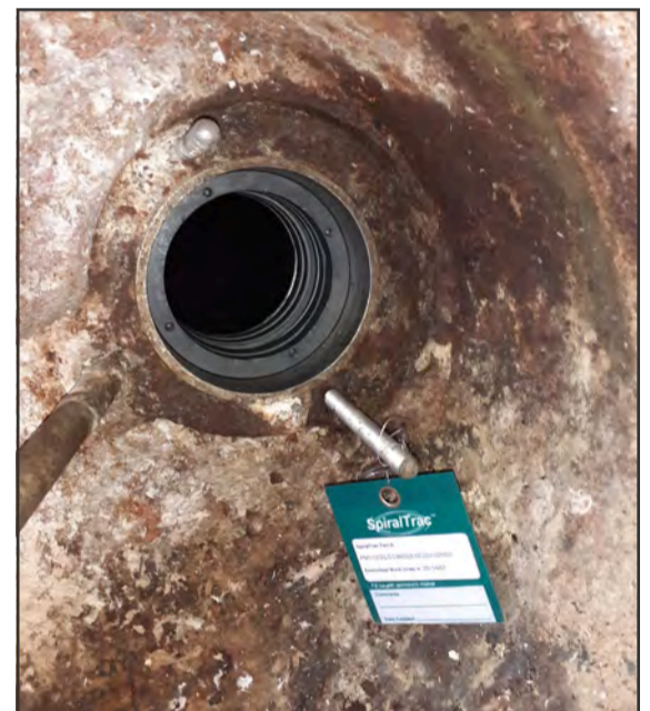
SpiralTrac being installed, green tag attached to equipment
