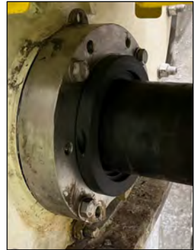
Spiraltrac Adaptor installed in cavity
