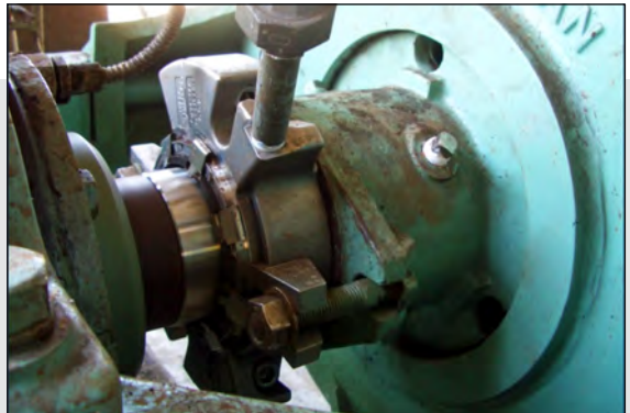
Chesterton solution being installed
