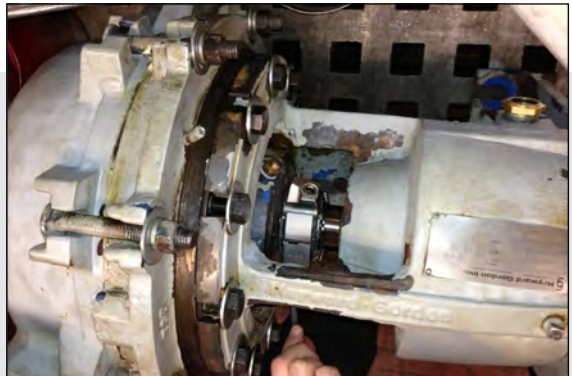
Chesterton solution being installed
