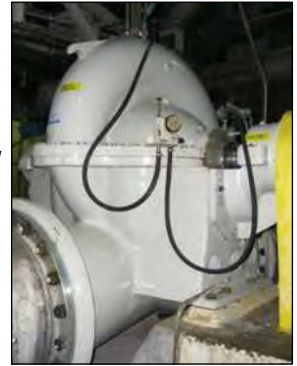
Chesterton Solution installed in Fan Pump
