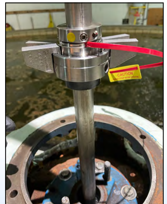
155 Seal being installed
