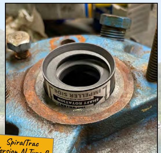
155 Seal being installed
