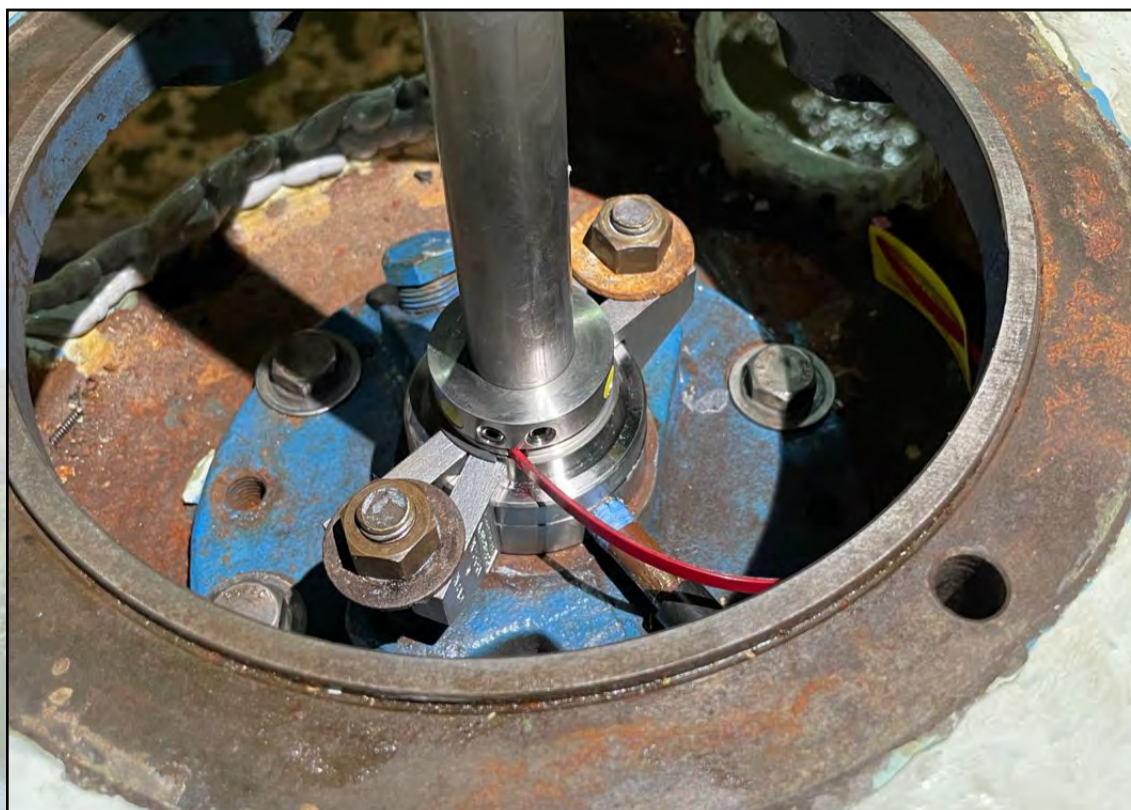
Chesterton Solution Installed
