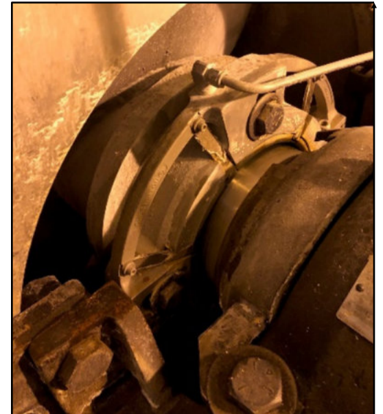
442 Split Seal installed
