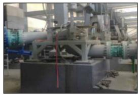
Dirt around the pump shows failure of original OEM dual seal
