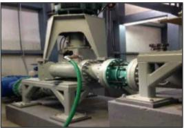
Pump area is leak-free with 442 and SpiralTrac installed
