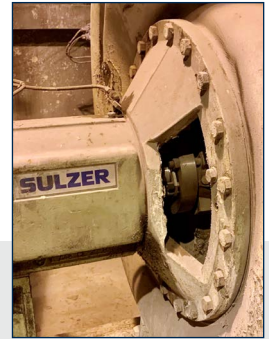
Zero leakage two years after installation of 170 Seal and SpiralTrac
