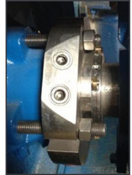
Chesterton S10 Cassette Seal installed in a Worthington Slurry Pump
