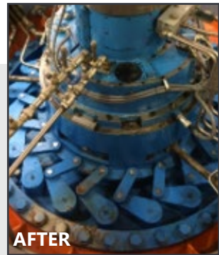
Turbine running leak free after 442 and Spiraltrac Adaptor installation
