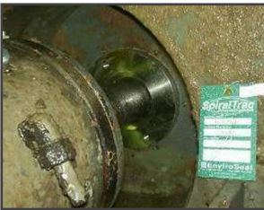
SpiralTrac Adaptor installed with green SpiralTrac tag
