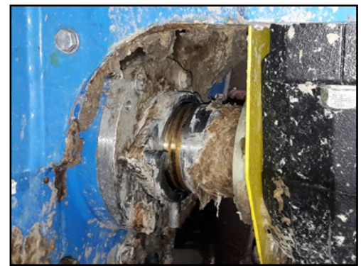
Before: a mixture of water and pulp in excessive flush leakage
