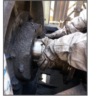
Chesterton SuperSet Being Installed
