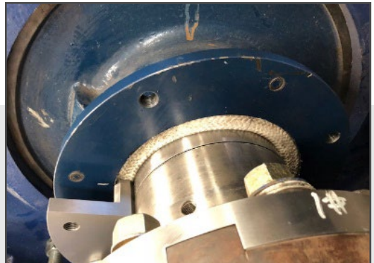
Installing Chesterton 1730 Mill Pack Packing
