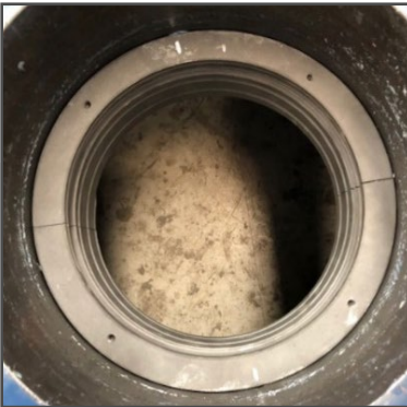
Installing Packing Version SpiralTrac
