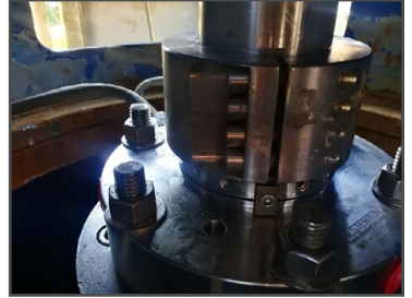
Linatex Slurry Pump with Chesterton Solution (180 seal and SpiralTrac) installed
