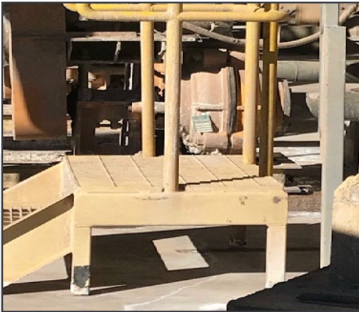
EnviroSeal green tag attached to pump with installed SpiralTrac information
